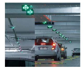
Fig. 1. Parking guidance system and occupancy sensors (Source: Siemens)
